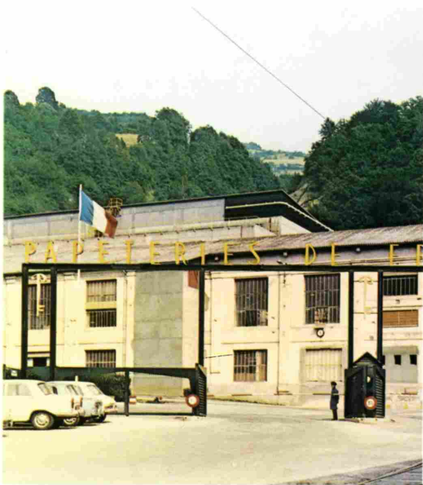
Recent major installation in a French paper mill typifies growth of international markets.
