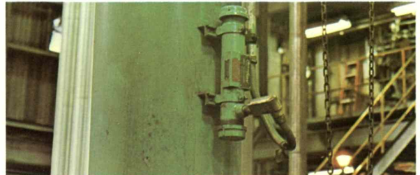
Density and level applications of AccuRay systems are common in the power industry.
