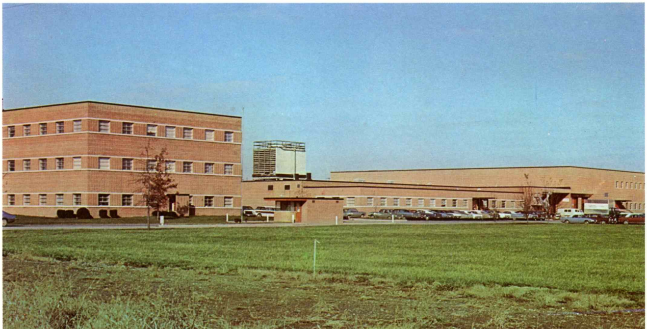
During the third quarter, a 71,000-square-foot, two-story addition for manufacturing and engineering enlarged the Ackerman Road headquarters to over 200,000 square feet.
